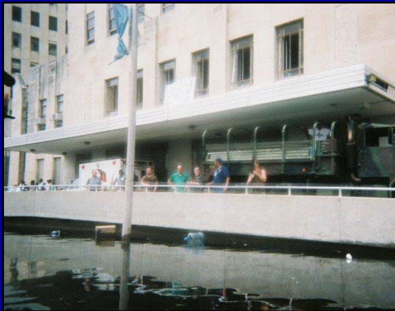
Charity Hospital ER Ramp
